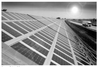
*Source: Fritta, S.L.* Fig. 10.- Panel of porcelain tiles fitted with photovoltaic cells
